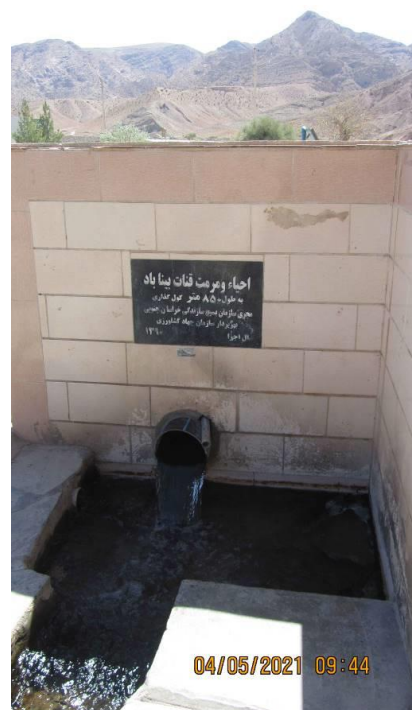
Figure 4. Qanat repairing and reconstructing in Binabad village, 70 km distance to Birjand, south east of Iran. Qanat has major role for sustainable exploiting of groundwater resources in Iranian rural people Indigenous Knowledge (IK) (By author, spring 2021).
